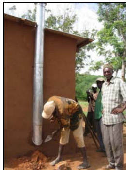
The chimney in place
