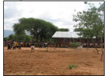
Chaludewa Primary School
