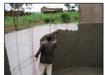
First layer of cement
