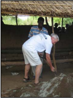
Mixing the cement
