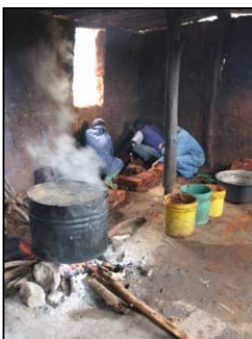
Old stove and new under construction
