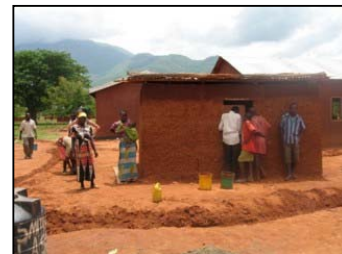
The new kitchen building
