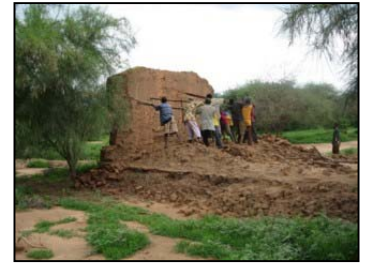
The collapsed building
