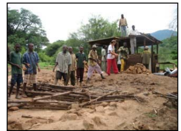
Re-using old bricks
